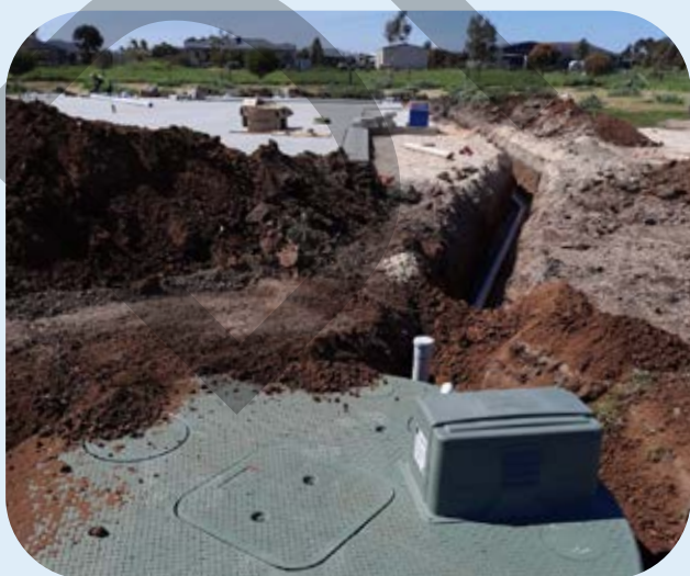
Aerobic wastewater treatment tank installation
