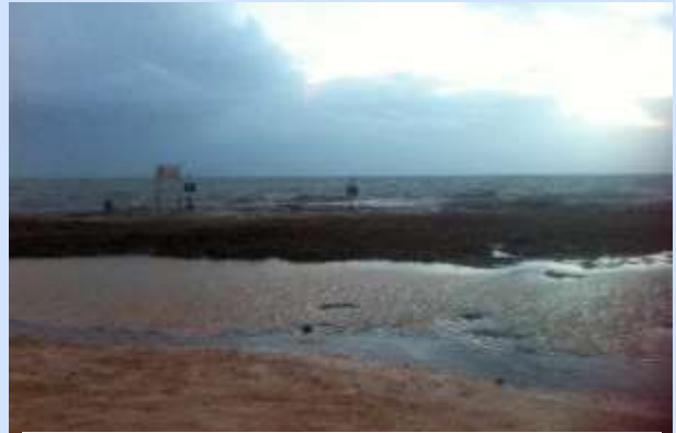
In some carparks, water flowed along the coast behind the front embankment / dune.
