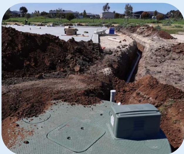
Aerobic wastewater treatment tank installation
