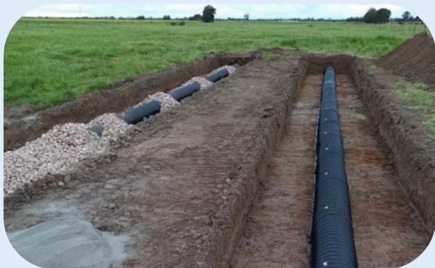
Septic soakage trench inspection
