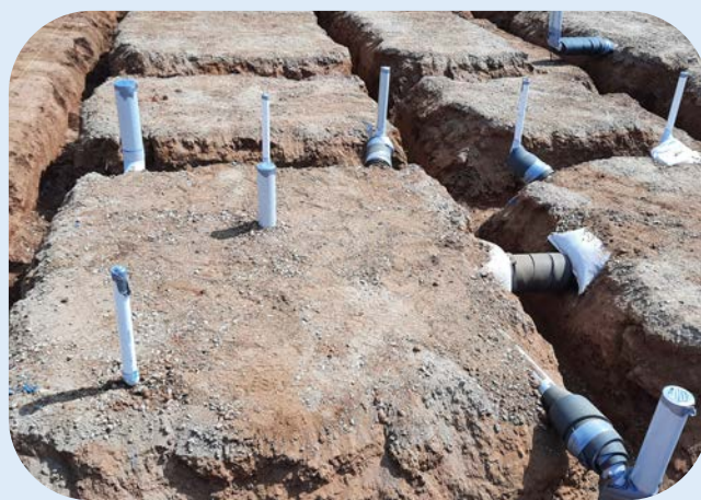
Underfloor plumbing inspection
