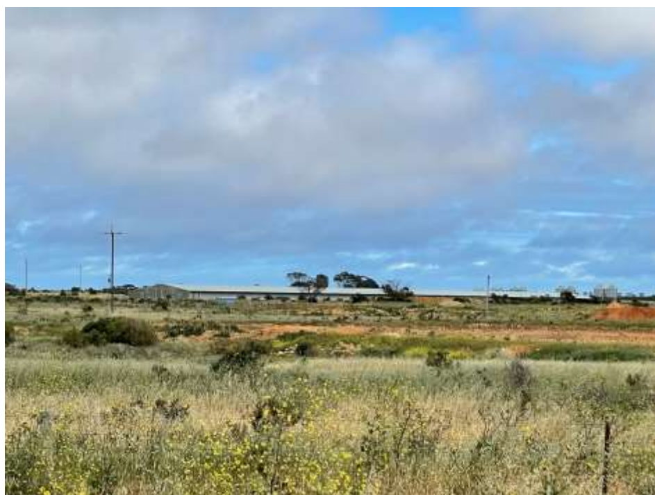
Figure 1: Subject land viewed from Lemmey Road
