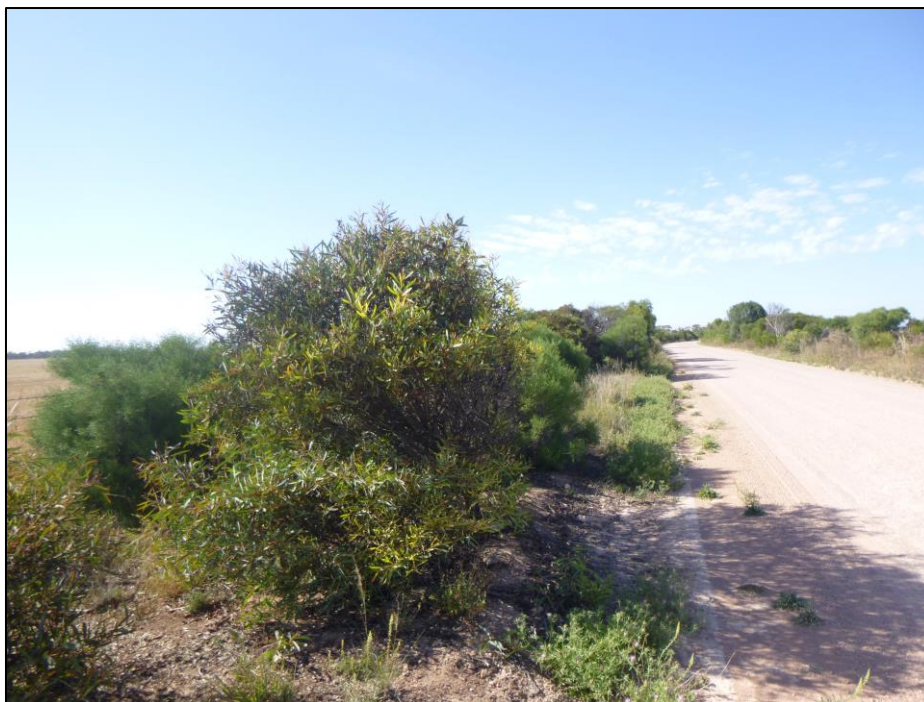
Figure 14. Example of clearance of regrowth required along the travelled way.
