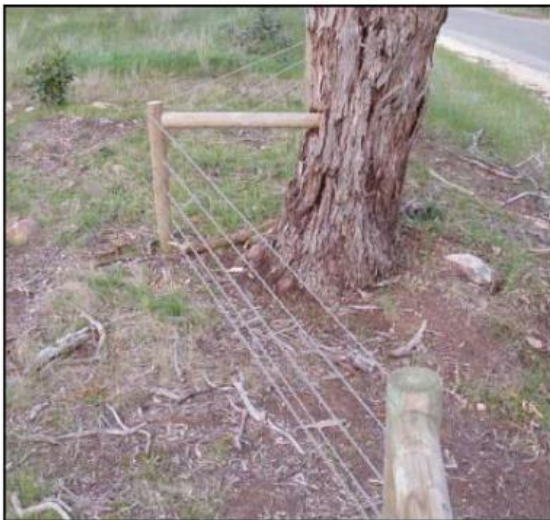
Figure 16. Simple strut arrangement that allows a fence to deviate a short distance around a large tree (NVC 2020b).
