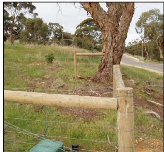
Figure 16. Simple strut arrangement that allows a fence to deviate a short distance around a large tree (NVC 2020b).
