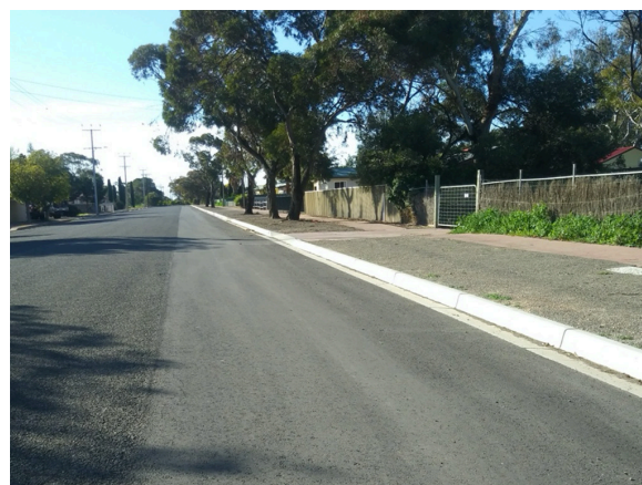
East side of Old Mallala Road Noble Crescent to North end – New kerb and shoulder seal
