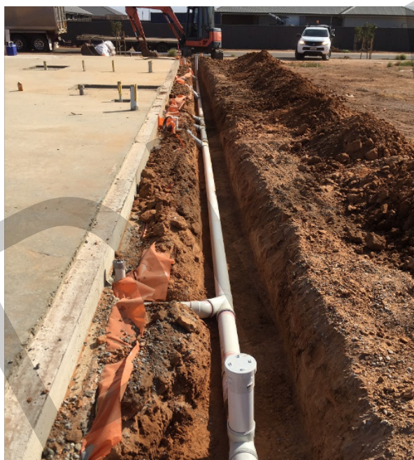
Inspections undertaken for installation of drains (left) and a pumping chamber (right) within the Eden Development at Two Wells.
