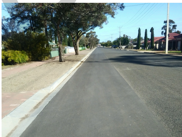
East side of Old Mallala Road Two Wells - Noble Crescent to North end – New kerb and shoulder seal
