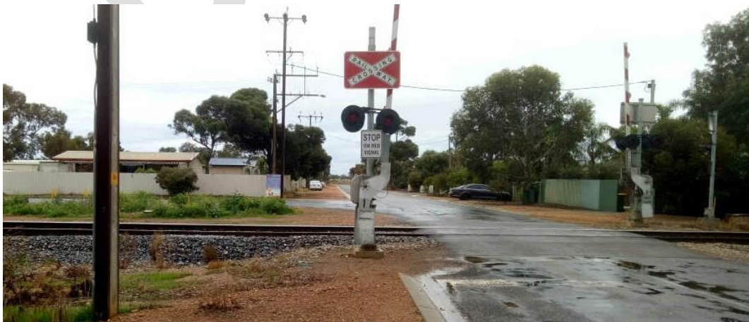
No formalised walking crossing exists at Elizabeth Street 2021
