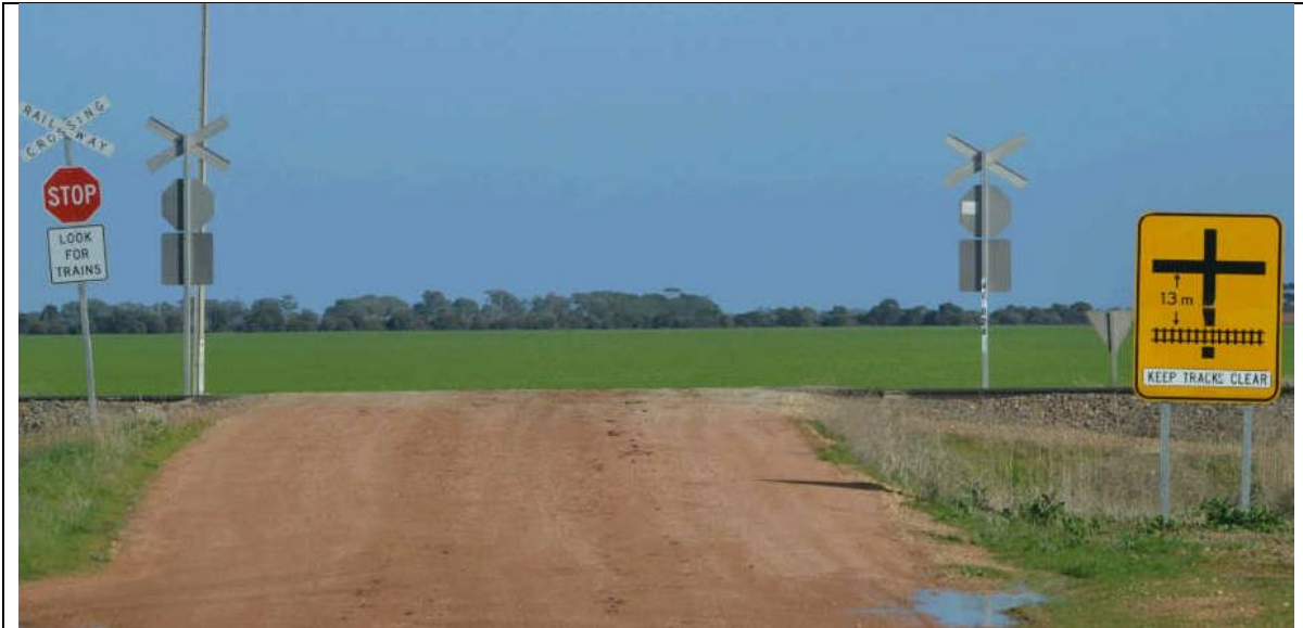
Temby Road crossing looking west July 2021. 13m from train line to Mallala Road provides limited vehicle space
