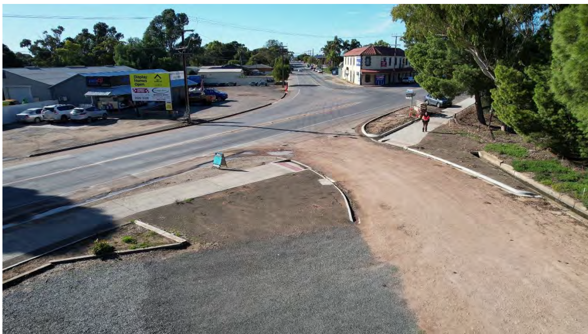
Figure 4 - Offset four-way intersection
