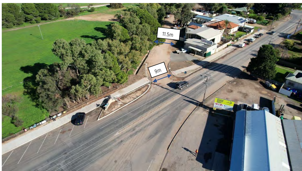
Figure 3 - Angled Windmill Road and Old Port Wakefield Road intersection to accommodate 19.1m refueling vehicle
