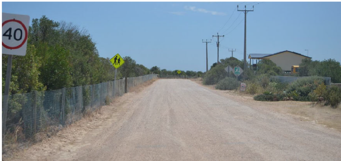
Figure 10 Council is investigating sealing the Esplanade
