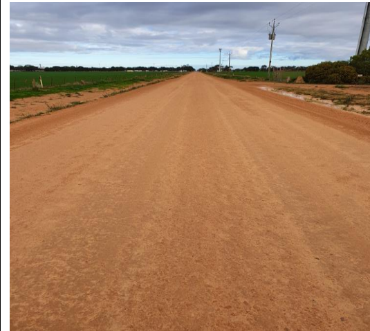
Typical Category 1 Road Rural Sheeted Road – Good Condition
