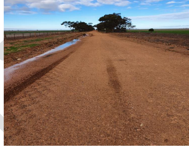
Typical Category 3-A Road Rural Sheeted Road Showing Signs of Wear and Developing of Patches
