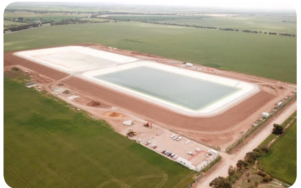
NAIS Storage Dam, Porter Road Korunye.
